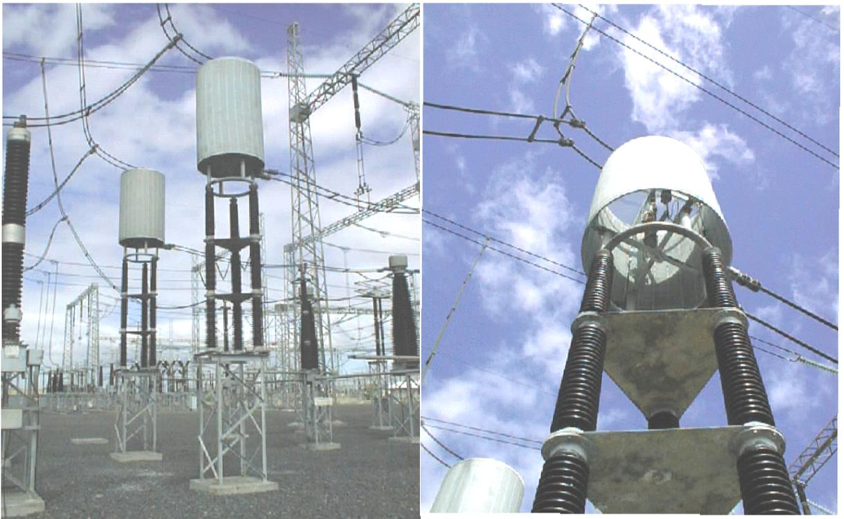
*Fig. 1.24: Typical Line Traps*
